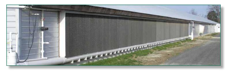
80, there is too much moisture in the air, and not enough holding capacity to effectively evaporate the moisture from the system, as well as the moisture created by livestock. However, when it's above 80, the air is usually dry enough to evaporate the water in the air, and the moisture from the house, meaning cooler conditions and dry litter. If the cool pads can be controlled via an Rh sensor the times of day can be ignored and pads set to only run when the Rh is below 80%.
