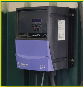
VFD Controls for variable speed operation
