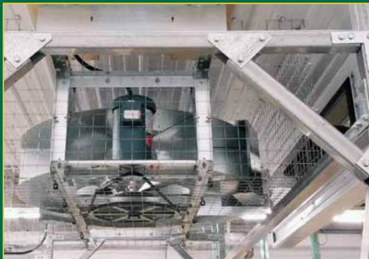
The Directional Hemisphere uses a shroud to divert mixing air from the Hemisphere away from the sidewall, working in concert with sidewall inlets.
