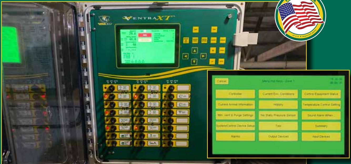
The Ventra XT incorporates a large 7" touch screen with a backlit display activated by a built-in proximity sensor.
