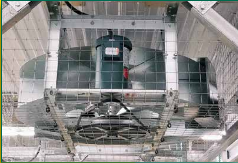
The shroud on the Directional Hemisphere helps circulate sidewall inlet air throughout the house.
