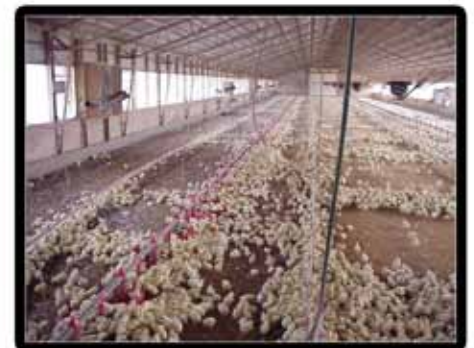
High intensity pancake heaters can produce hot spots creating uneven heat patterns causing birds to bunch together seeking comfort zones.
