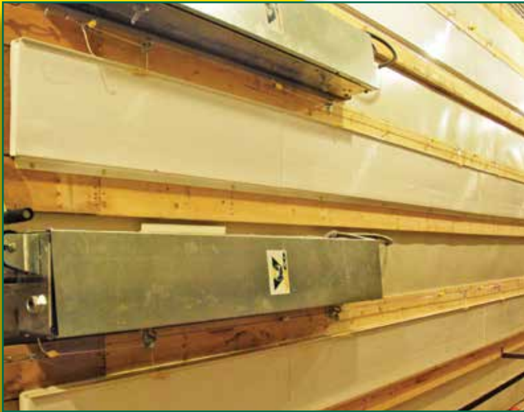
Continuous inlets are designed to run the entire length of the house.
